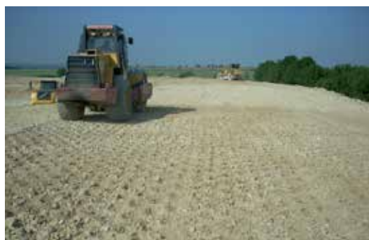
Picture 33: Compaction of the embankments with chevron tamping wheels compactor
