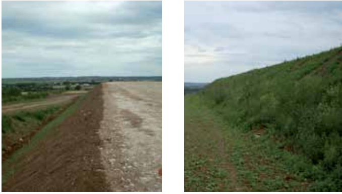
Figure 23: External embankment (before and after seeding)
