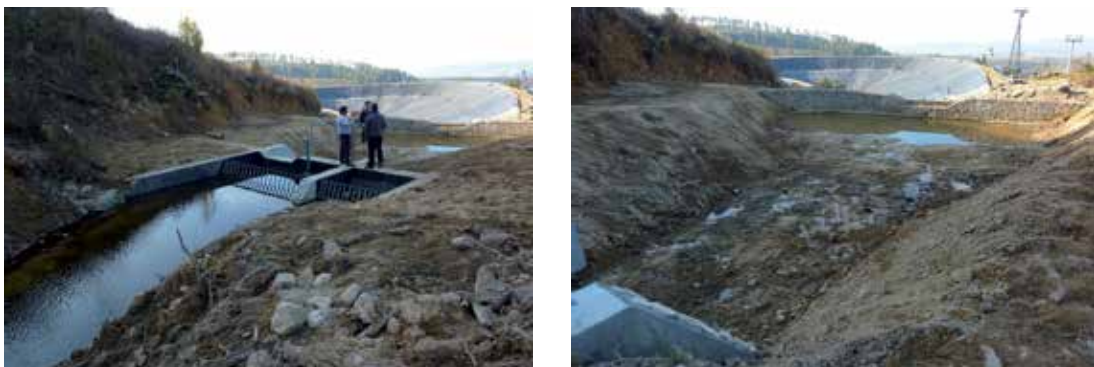
Picture 214: Hydraulic infrastructures upstream (river bed) to remove sediments and floating objects and for the bypass
