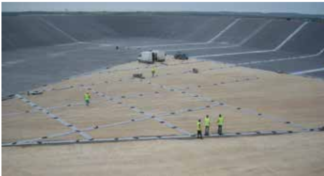
Figure 28: Gas drainage with geocomposite
