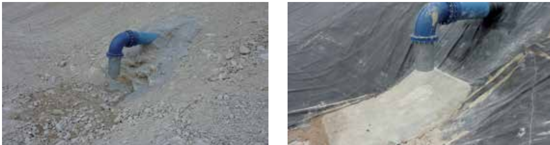
Picture 216: Water outlet pipe in the embankment with ballasting concrete slab
