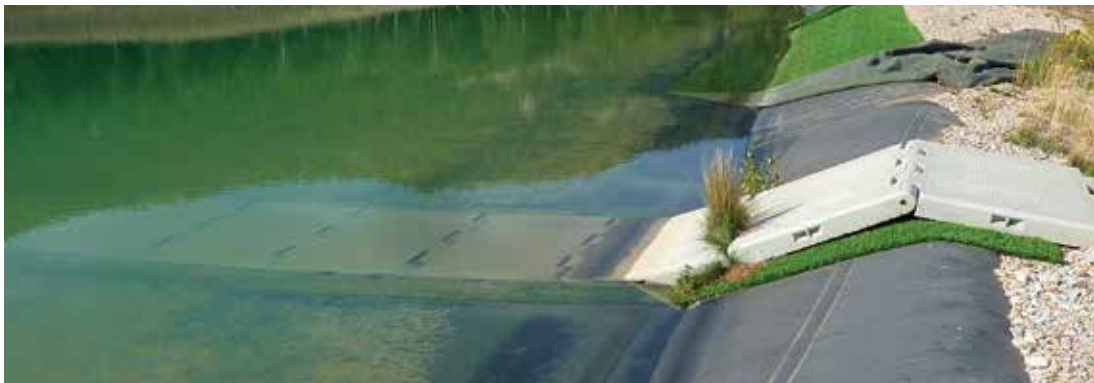
Picture 224: Wind ballast with precast concrete slabs anchored on the crest
