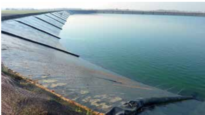
Figure 38: Wind ballast with PE bags filled with gravel and anchored on the crest
