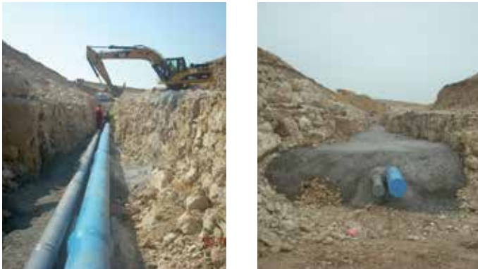
Figure 24: Outlet and water drainage pipes through the embankment
