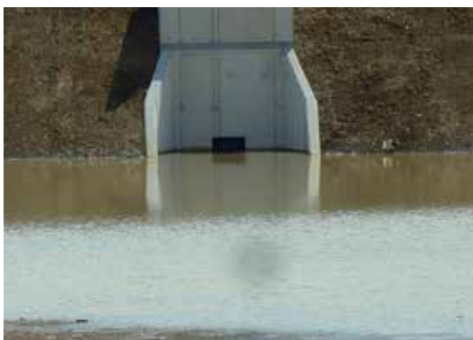
Picture 218: Concrete water outlet combined with the spillway
