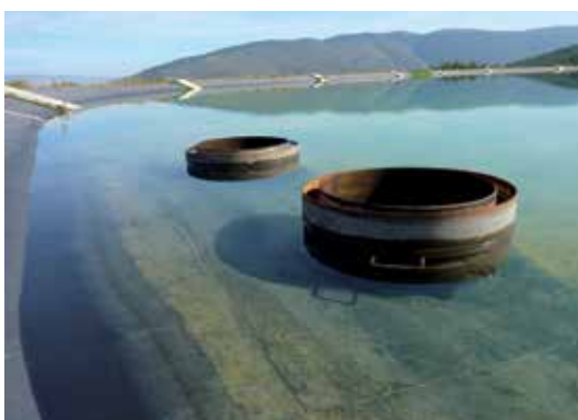
Picture 222: Pipe spillway
