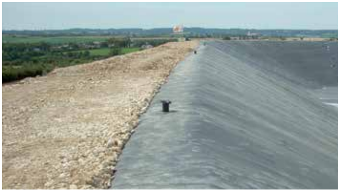
Figure 36: Anchor trench after back filling
