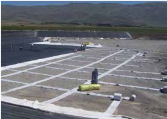
Picture 26: Gas drainage with geocomposite
