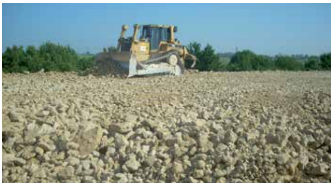
Figure 16: Leveling with bulldozer on the embankments
