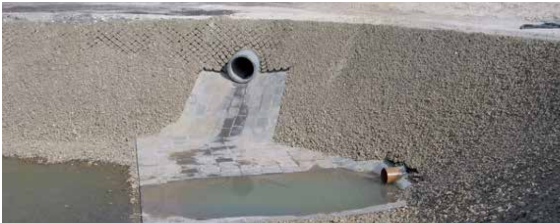
Picture 213: Pipe water inlet with covered embankments
