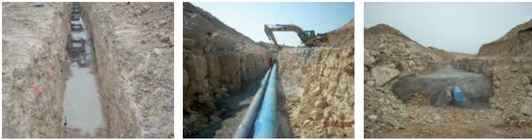
Picture 215: Outlet pipe through the embankment
