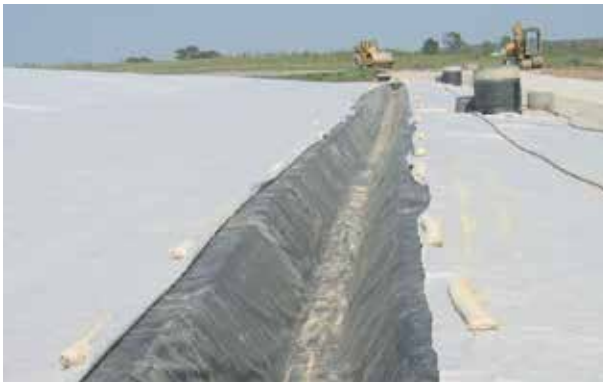
Figure 7: Installation of the peripheral ditch and high protection geotextile
