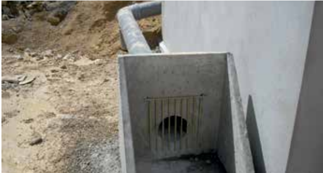
Figure 27: Water drainage outlet
