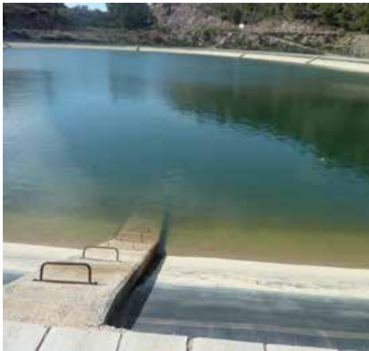
Picture 226: Wind ballast with precast concrete running on the entire slope
