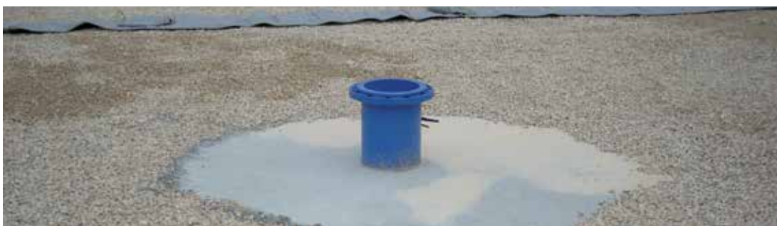
Picture 219: Good quality concrete structure around water outlet pipe
