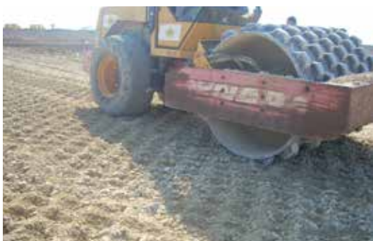
Picture 33: Compaction of the embankments with chevron tamping wheels compactor
