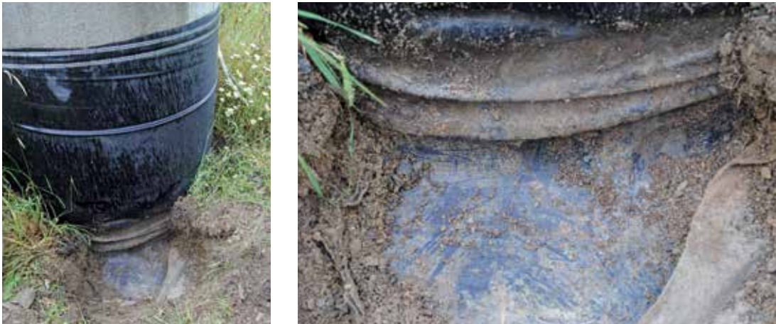
Figure 18: Degassing well – inspection of connection detail
