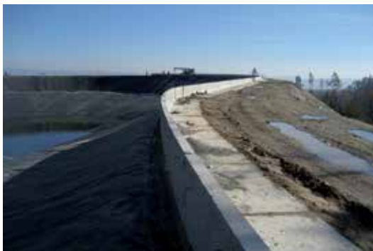
Picture 21: Extra protection on the crest against waves overflow
