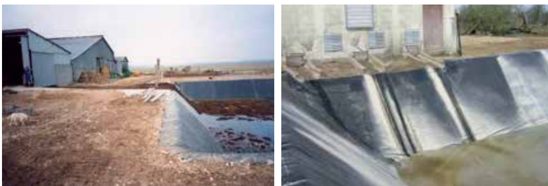
Photo 56: Direct filling of effluent
