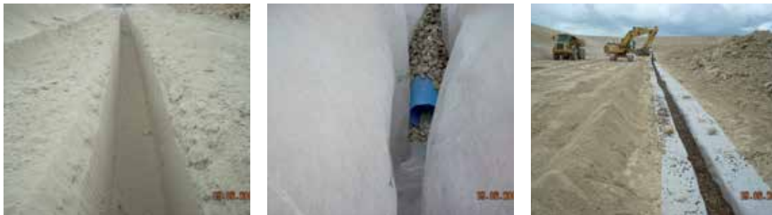
Picture 24: Drainage ditch
