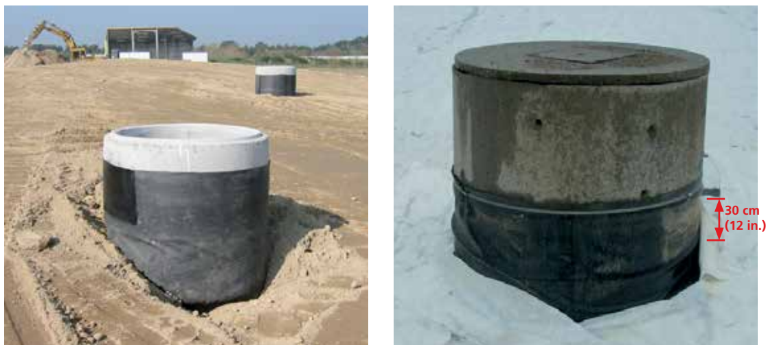
Figure 10: Degassing well before and after the addition of a safety pleat
