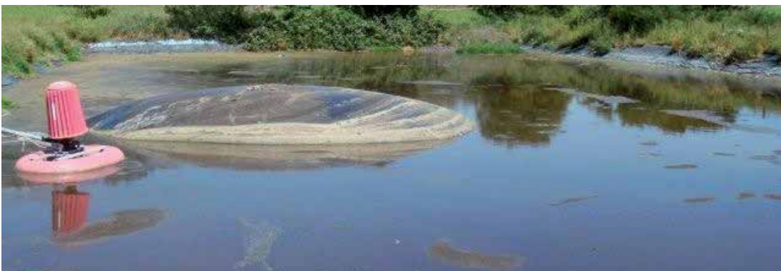
Picture 28: Gas trapped under the geomembrane
