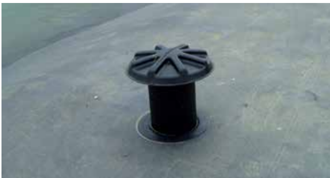
Figure 29: Gas vent at the top of the embankment
