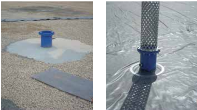
Figure 25: Water outlet pipe at the bottom
