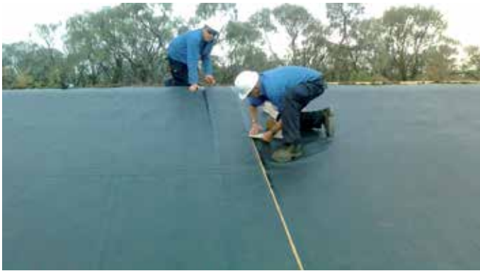
Figure 33: Seaming of EPDM geomembrane
