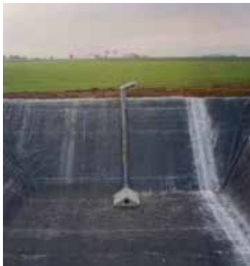
Photo 513: Pond outlet system (suction pumping)
