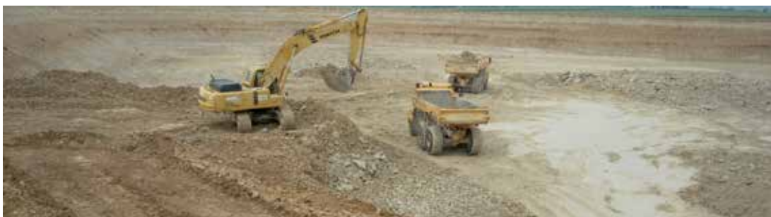
Picture 31: Excavation of the base of the pond and truck loading
