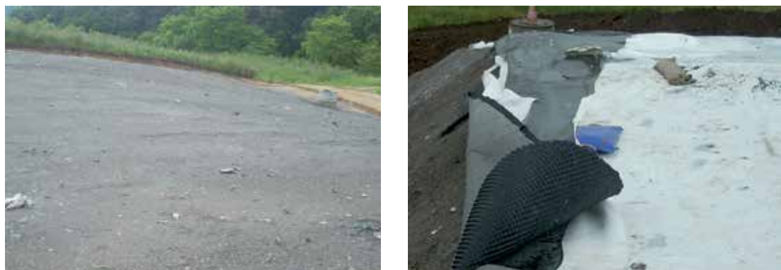
Figure 5: Reprofiling layer prior to installing the impermeable geomembrane system and gas drain geocomposite
