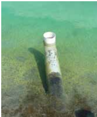
Figure 37: Pipe spillway
