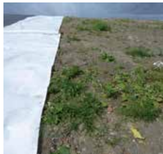
Picture 23: Unacceptable support layer
