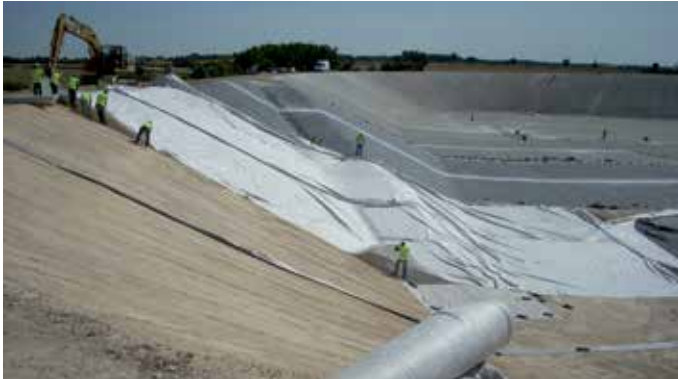
Figure 30: Geotextile installation
