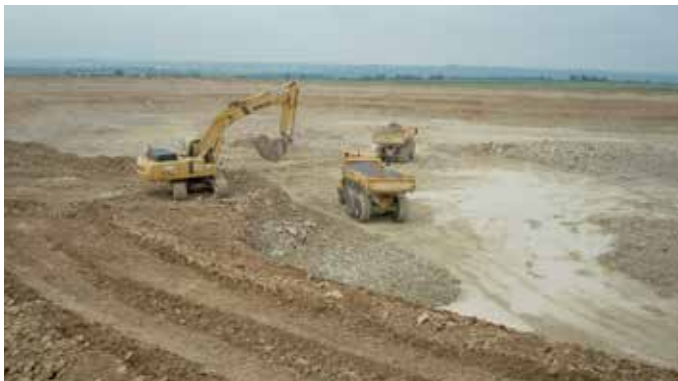
Figure 14: Excavation of the base of the pond and truck loading
