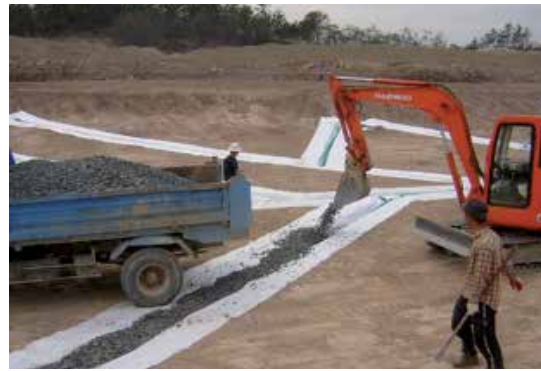
Photo 54: Filling of trenches with draining gravel
