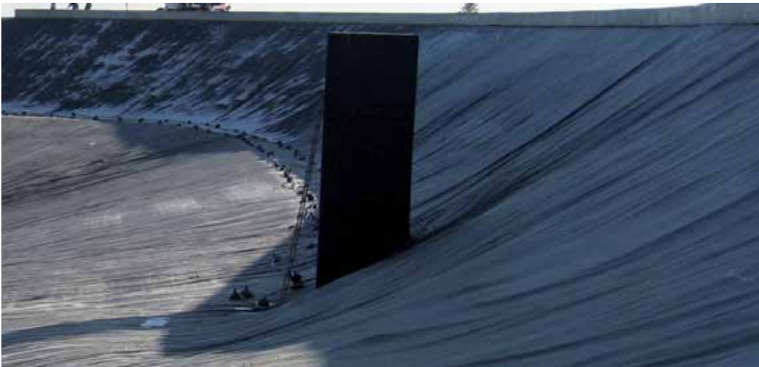
Picture 223: Spillway tower
