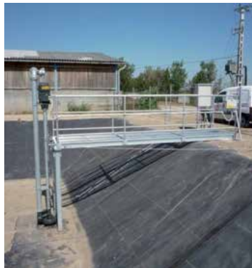
Photo 514: Pond drainage system (pressure pumping)
