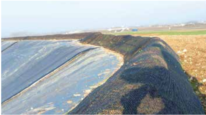
Figure 39: Waves protection
