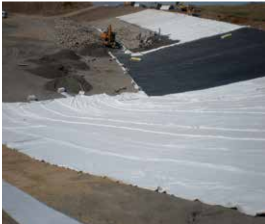
Picture 29: Riprap cover installation
