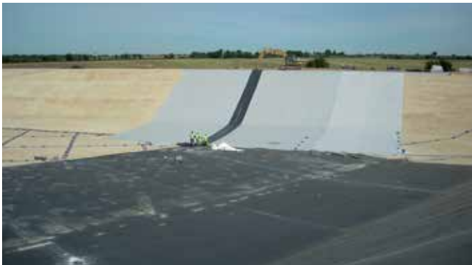
Figure 31: Unrolling of EPDM geomembrane
