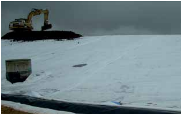
Figure 8: Installation of the soil cover
