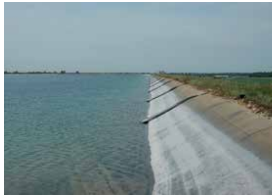
Picture 225: Wind ballast with PE bags filled with gravel and anchored on the crest
