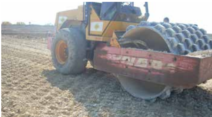
Figure 17: Compaction of the embankments with chevron tamping wheels compactor
