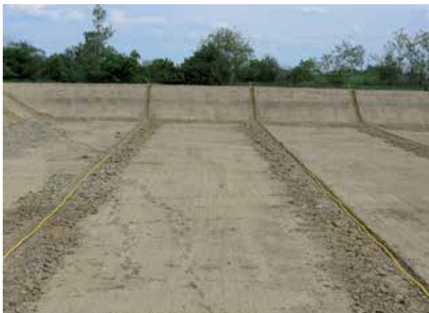
Picture 25: Gas drainage with pipes
