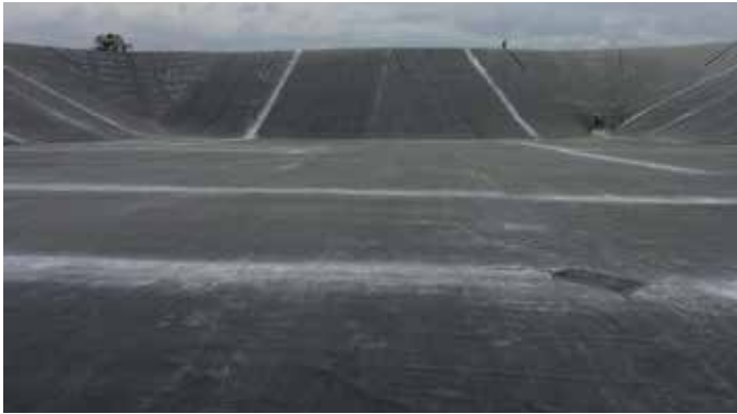
Figure 34: Installed EPDM geomembrane
