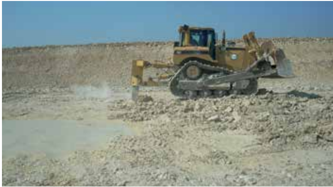
Figure 11: Rock breaking at the base of the pond
