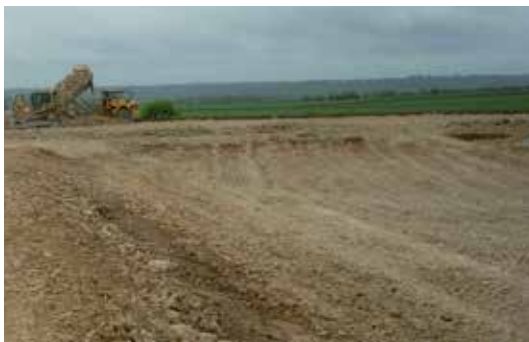
Picture 32: Unloading of excavated ground and levelling with bulldozer on the embankments
