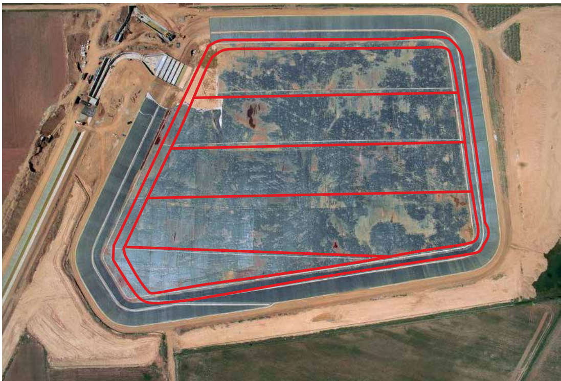
Picture 227: Wind ballast with precast concrete on intermediate berm, at the toe of the slope and the bottom surface
