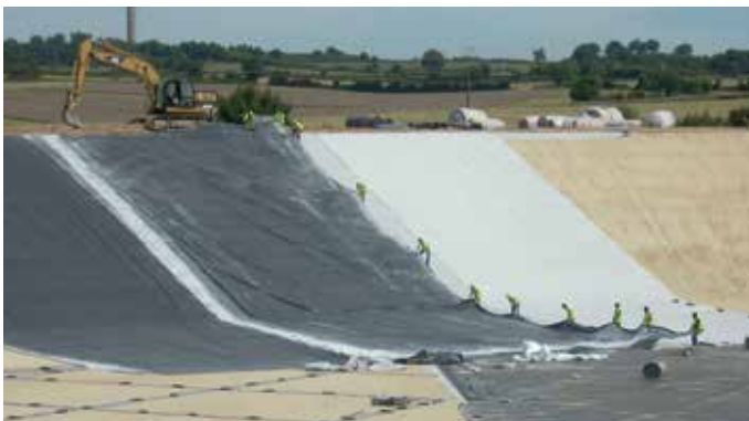
Figure 32: Unfolding of EPDM geomembrane
