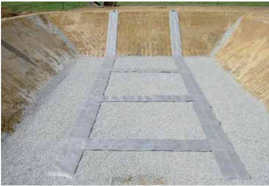
Photo 59: Gas drainage network (geocomposite) + draining layer of 10 cm (4 in.)
