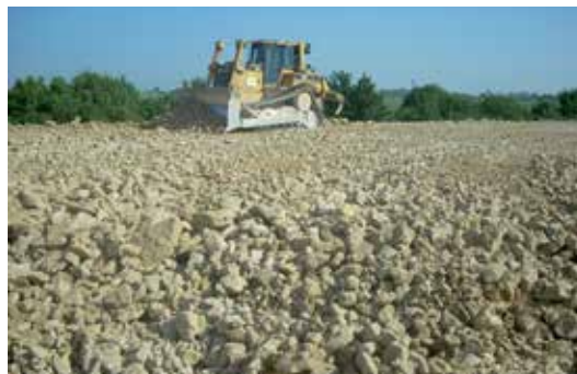
Picture 32: Unloading of excavated ground and levelling with bulldozer on the embankments
