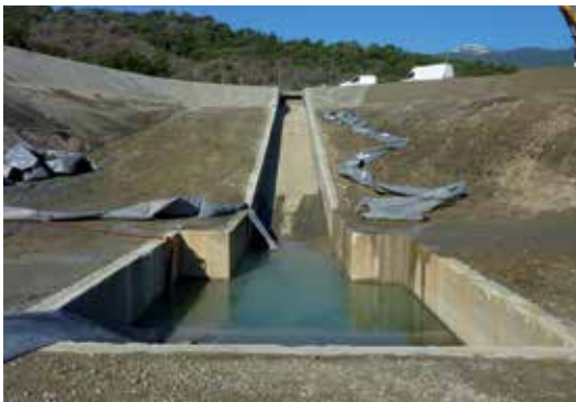
Picture 211: Concrete water inlet from the top of the embankment
