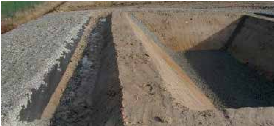
Photo 58: Anchoring trenches
