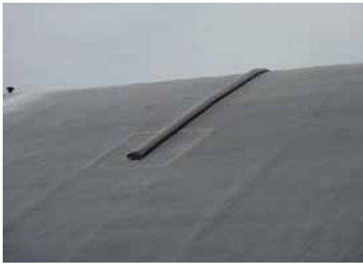
Picture 225: Wind ballast with PE bags filled with gravel and anchored on the crest
