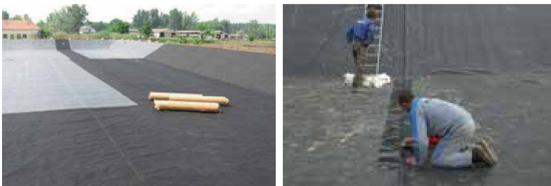
Photo 512: Installation and assembly of the geomembrane
