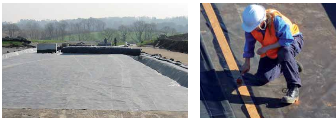
Figure 6: Installation of the EPDM geomembrane. Creating a seal using self-adhesive tape
