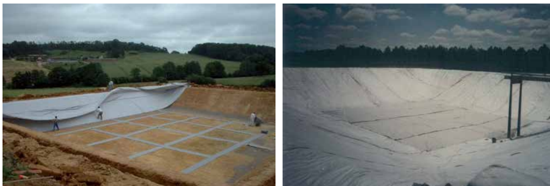
Photo 511: Installation of the geotextile
