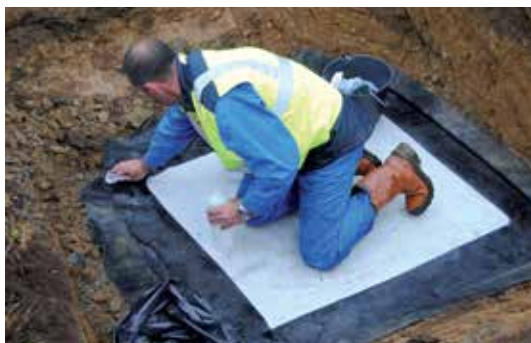
Figure 13: Cleaning and repairing the EPDM geomembrane
