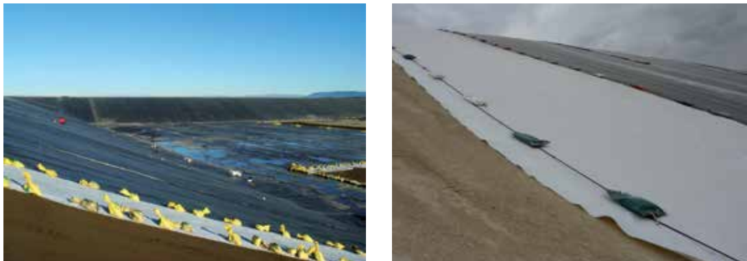
Picture 313: Temporary ballast of the geotextile and the geomembrane with sand bags
