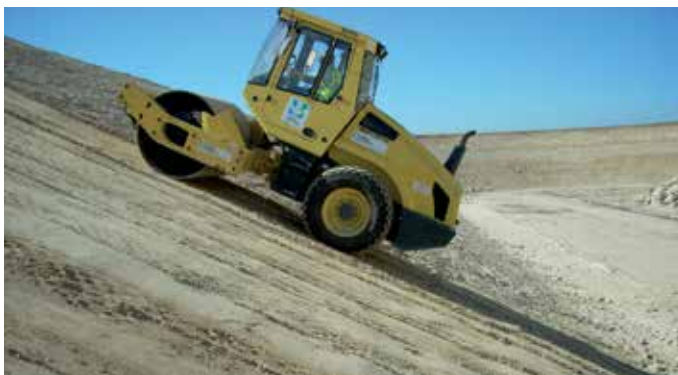
Figure 21: Final compaction
