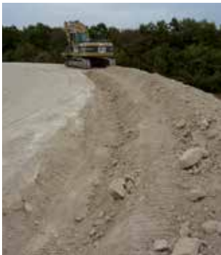
Figure 35: Anchor trench with geotextile
