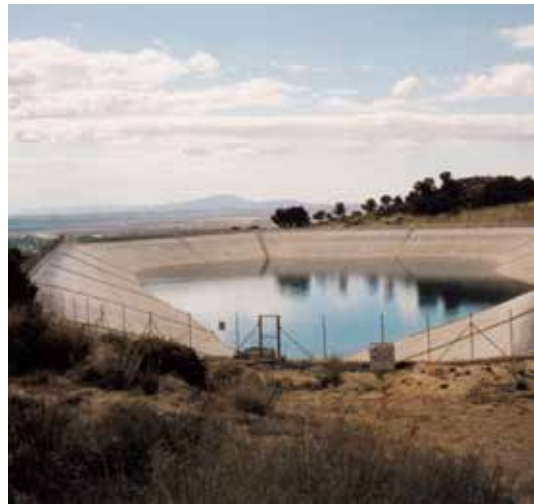
Picture 225: Wind ballast with PE bags filled with gravel and anchored on the crest
