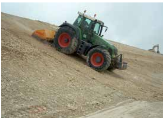
Picture 37: Stone crusher and final compaction
