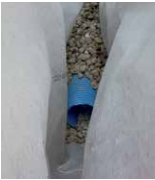
Figure 26: Water drainage ditch
