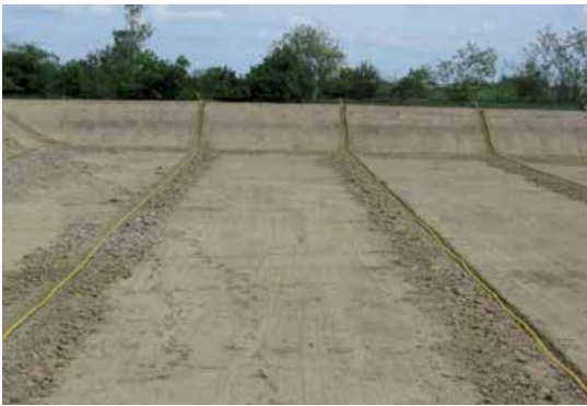
Photo 510: Gas drainage network, (perforated pipes)
