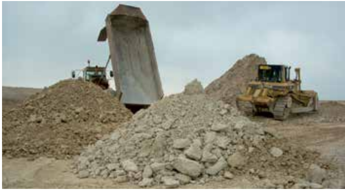
Figure 15: Unloading of excavated ground on the embankments
