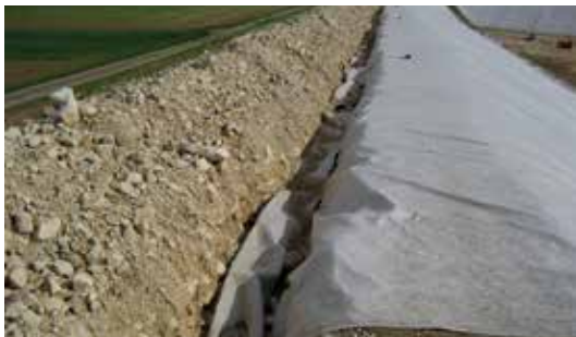
Picture 39: Anchor trench with geotextile before and after back filling
