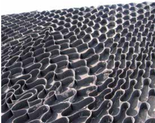
Picture 210: Cellular geogrids filled with cover material
