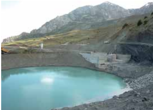
Picture 220: Free weir spillway upstream
