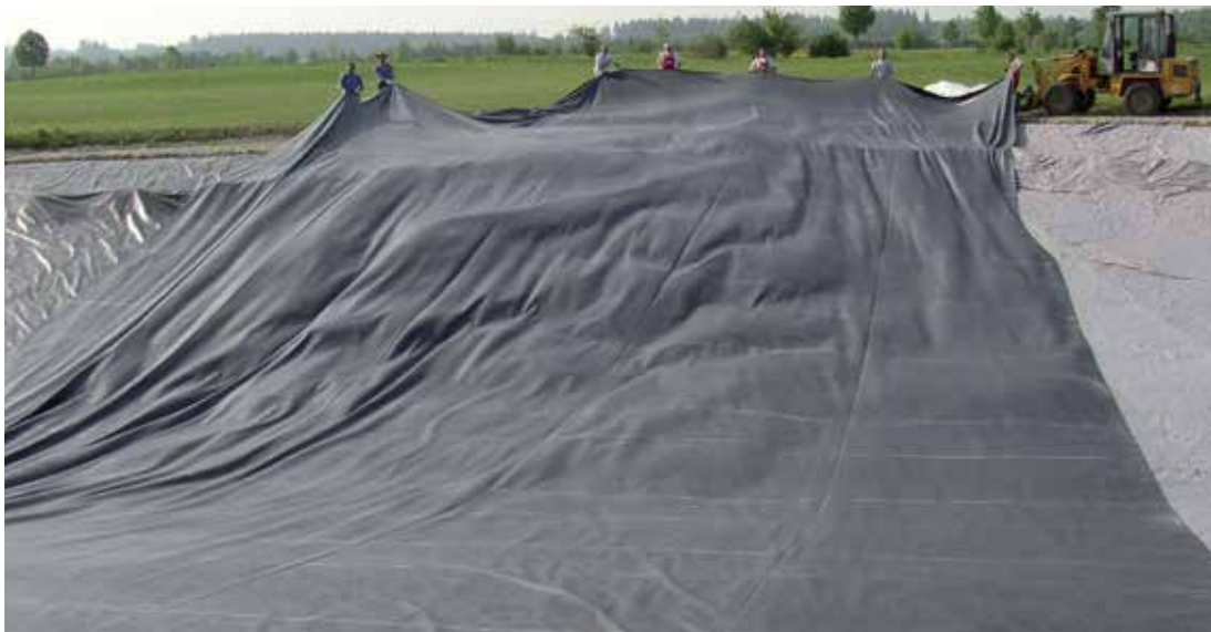
Picture 312: Moving the geomembrane on air cushion
