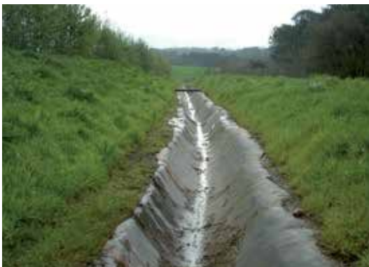
Figure 3: Peripheral ditch at the foot of the mound lined with EPDM geomembrane
