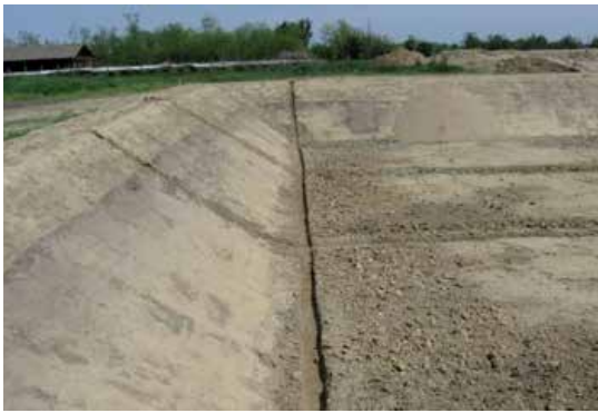
Photo 53: Trench for the peripheral drain at the foot of the embankment
